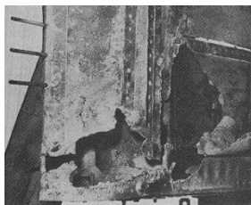
Figure 2. Damage caused by heat concentration due to shockwave impingement at a boundary layer during a X-15 flight. (NASA)
