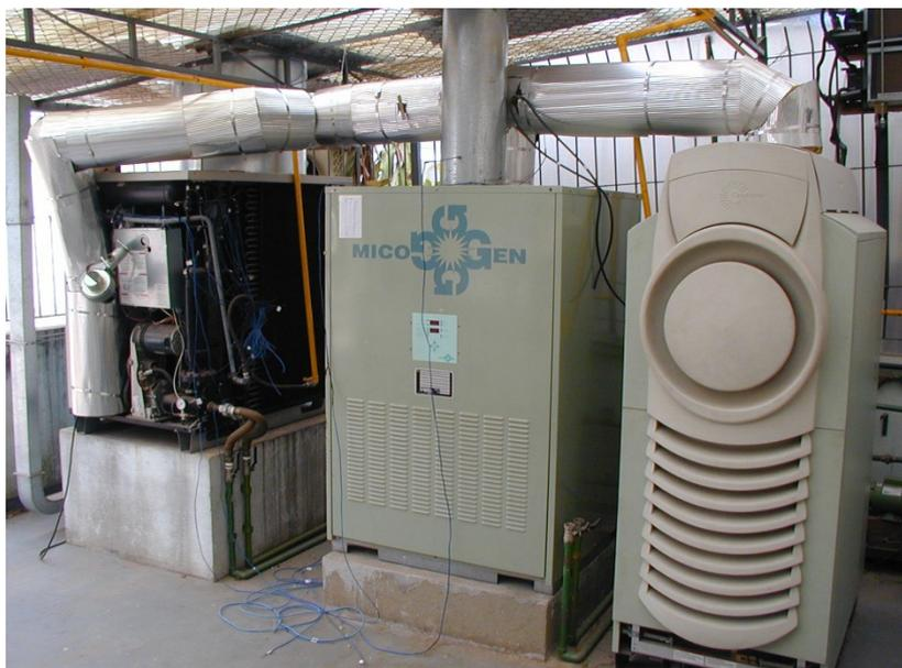
**Figure 2.** Trigeneration system view.
