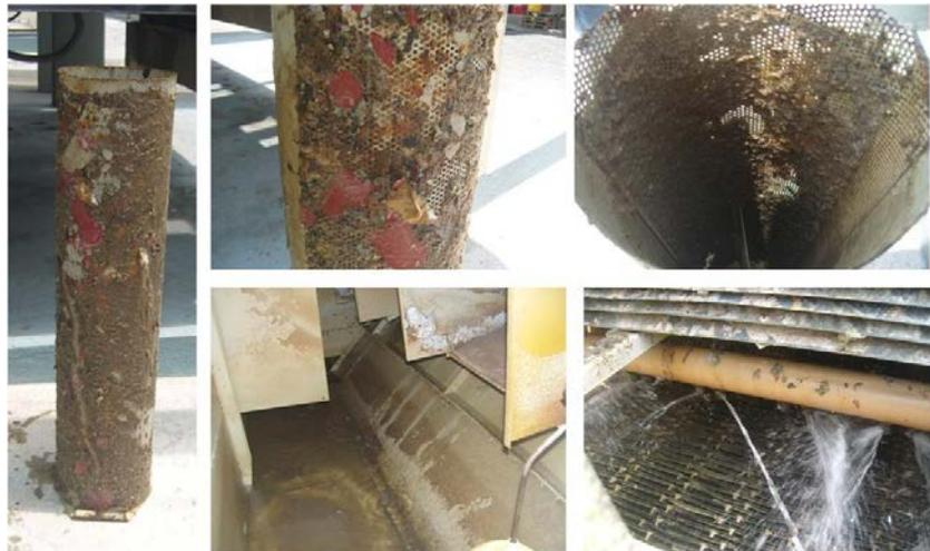
Figure 3. Clogging of filters and spray nozzles of the cooling towers
