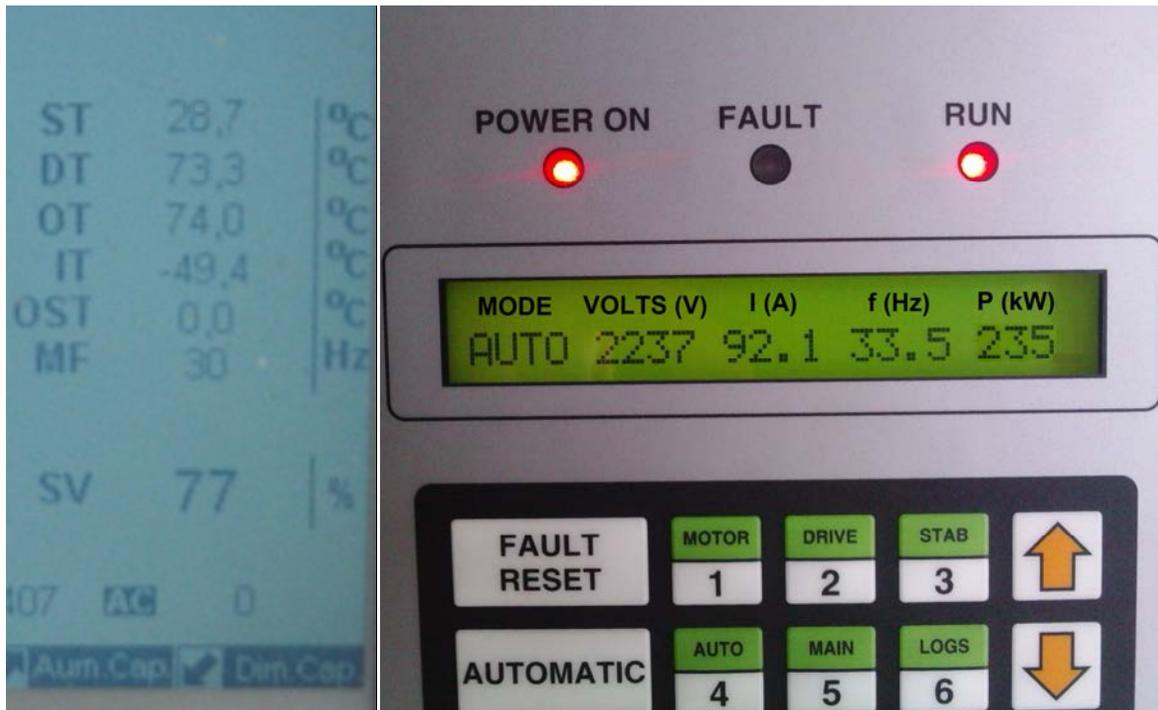
Figure 7. Dates of screw compressor modulating with VSD
