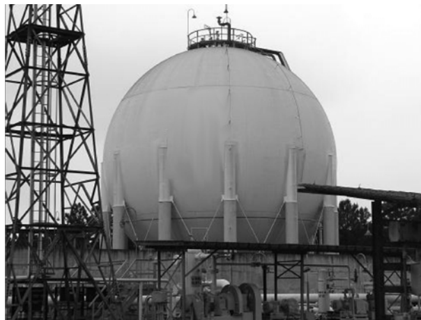
Figure 1. LPG storage sphere.
