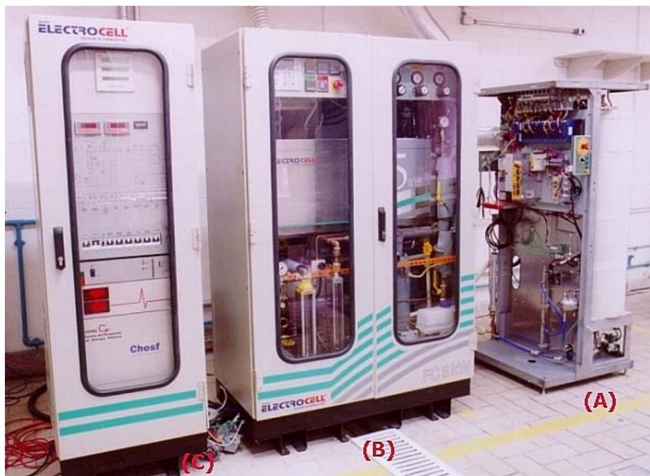
Figure 9. PEMFC system installed at CEPEL's laboratory: (A) Natural gas reformer; (B) Fuel cell unit and (C) Power conditioner (Serra et al., 2005).
