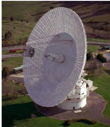
Figure 1 – Deep Space Network (DSN) 70 m diameter antenna, in Canberra/Australia.
