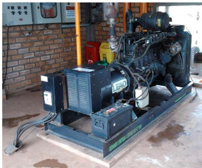
Figure 2. MWM 6.12T Gas Engine
