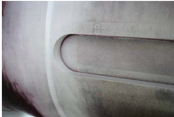
Figure 10. Shaft inspection using the penetrated liquid test
