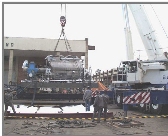
Figure 5. Expander being transported to the FCC unit
