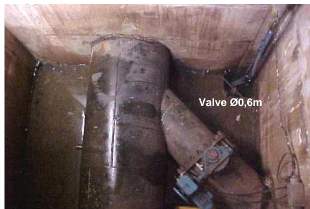
Figure 3. Valve's well for the connection of the auxiliary water intake conducts
